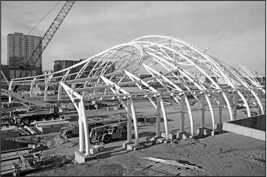
The shape of the framework for part of the new platform cover is seen from an upper window of the Denver depot. – Photo © 2012 Dave Schaaf.
