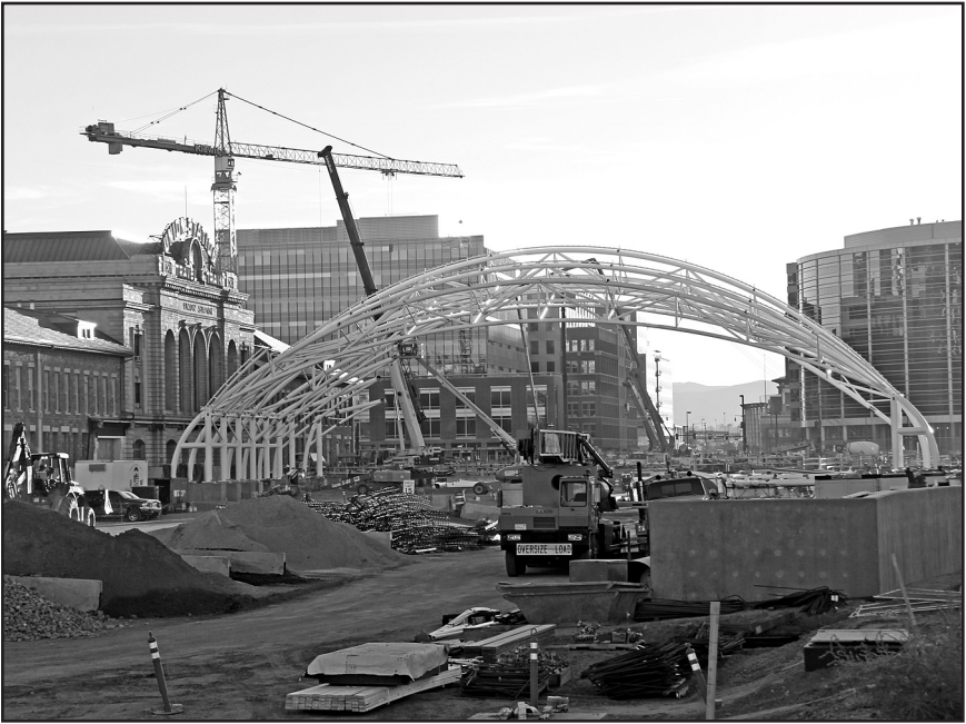
Construction of the canopy over the passenger tracks adjacent to Denver Union Station is underway on November 20, 2012. – Photo © 2012 Dave Schaaf.
